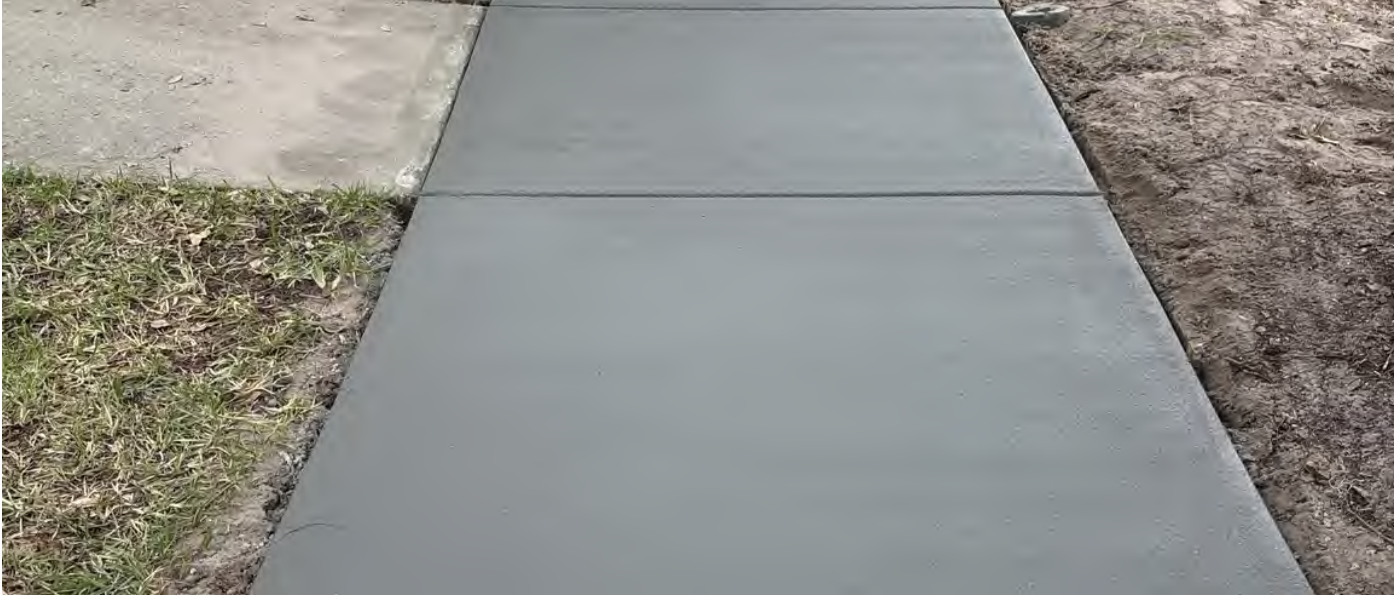
Representative site access condition - sidewalk setback and vegetated roadside drainage swale.
